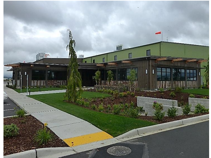
Skagit Valley Farm Cooling – new facility completed August 2019
