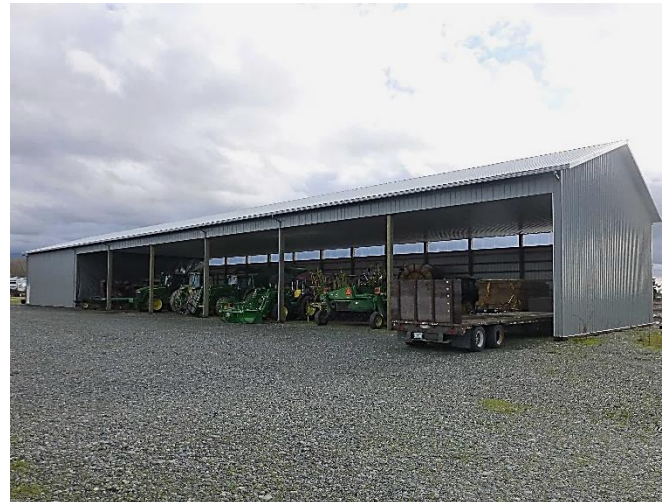
Residential agricultural building – completed January 2019
